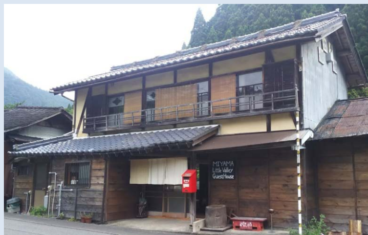
写真1-1 Miyama Little Valley Guest House
